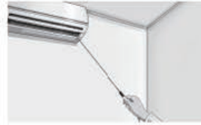
Temperature measurement of blowout hole of air-conditioner 空调出风口温度检测
